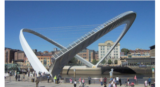
Millennium Bridge in Gateshead, England
